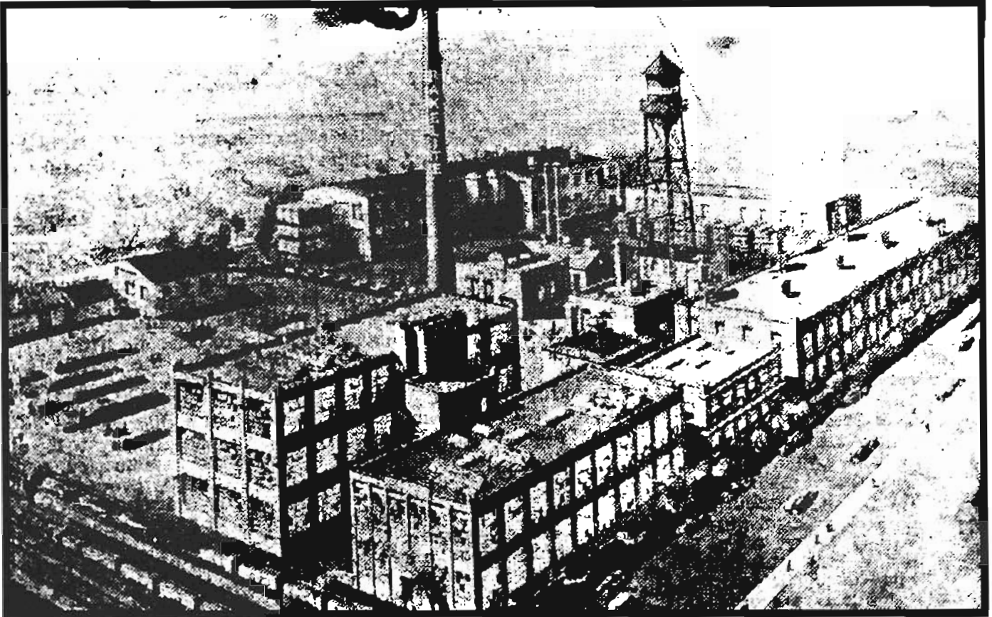
"Wash drawing" of Bakelite Plant in Bloomfield, N.J. 1940 ( Independent Press 1940). Grove Street is on the right, the Erie railroad tracks, now CONRAIL, can be seen in the lower left corner.
