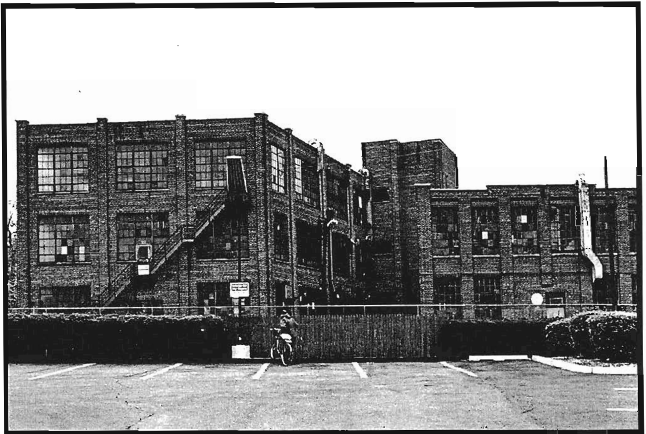
Southern facade of Bloomfield DPW facility buildings from adjacent parking lot of a Roy Rogers restaurant on Boomfield Avenue. These two buildings, erected between 1923 and 1928, were experimental labs in 1938 (see Figure 15). (March 12, 1996)
