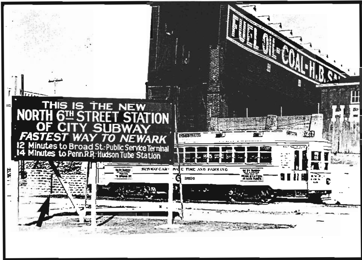
New North 6th Street Station on December 9, 1940 with Car 2616 serving as a waiting room. Note H.B. Salmon Co. Building also seen on Figures 26 and 27 (courtesy of John Catrambone). Note new stone wall (arrow).
