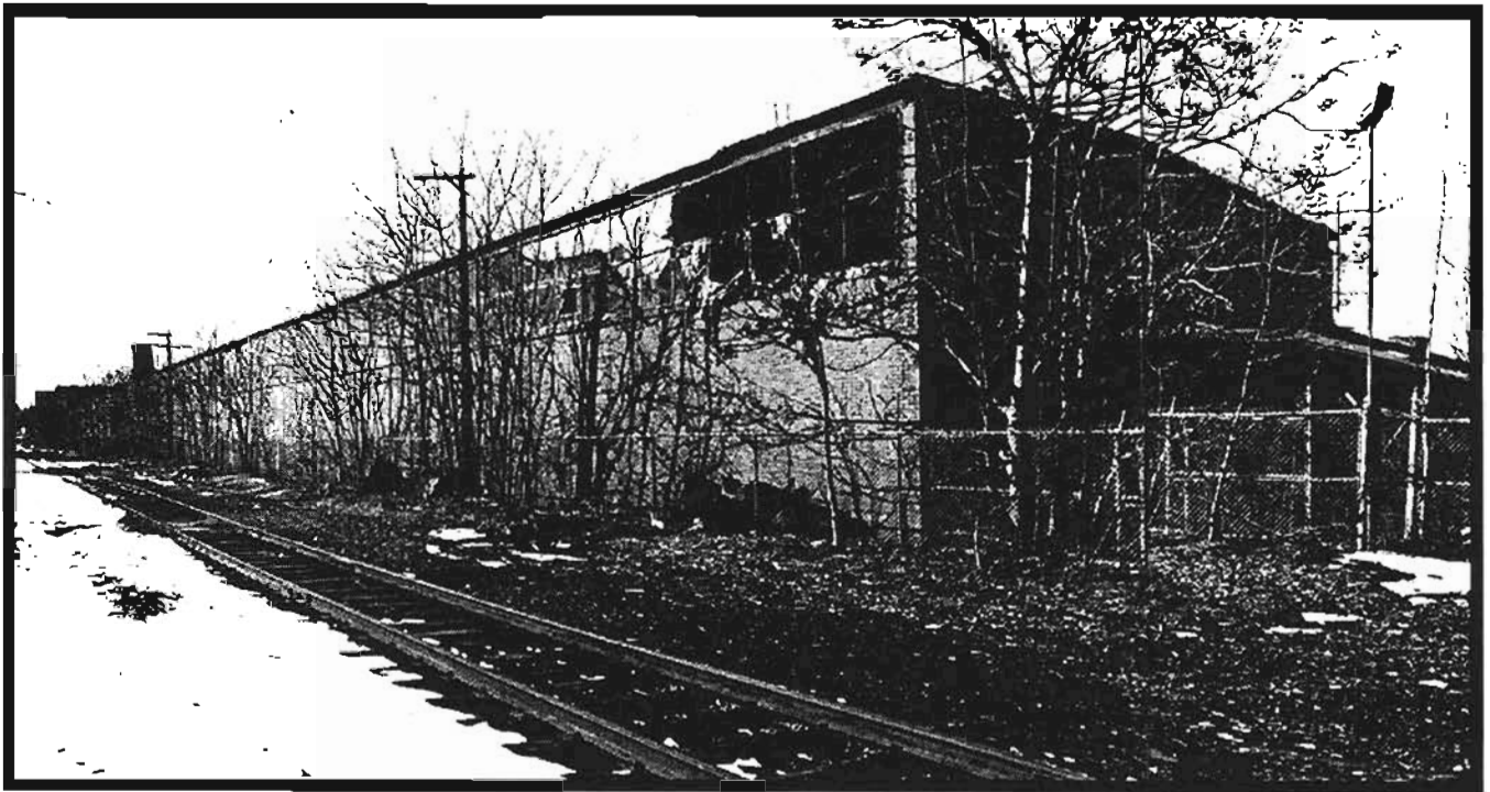
Composite view of abandoned Potamkin Cadillac Service and Parts building, the site of the VBF on north side of former CONRAIL tracks. View is west toward Grove Street. (March 12, 1996)
