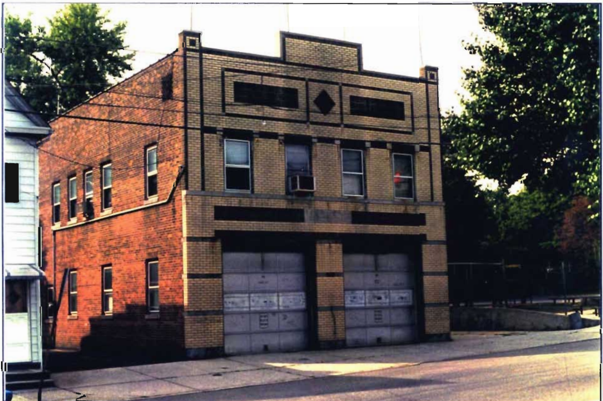
Photo F-2: Fire Station No. 1, Williams Street at Washington Place.
