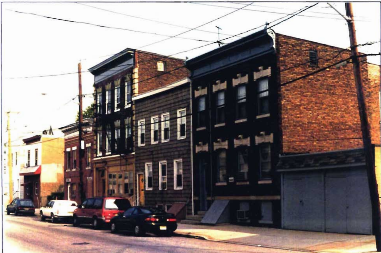
Photo B-2: South Side of Belmont Avenue (Opposite 41 Belmont Avenue)
