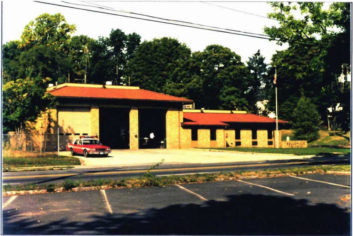
Photo F-1: Fire Department Headquarters Building, 275 Franklin Avenue.
