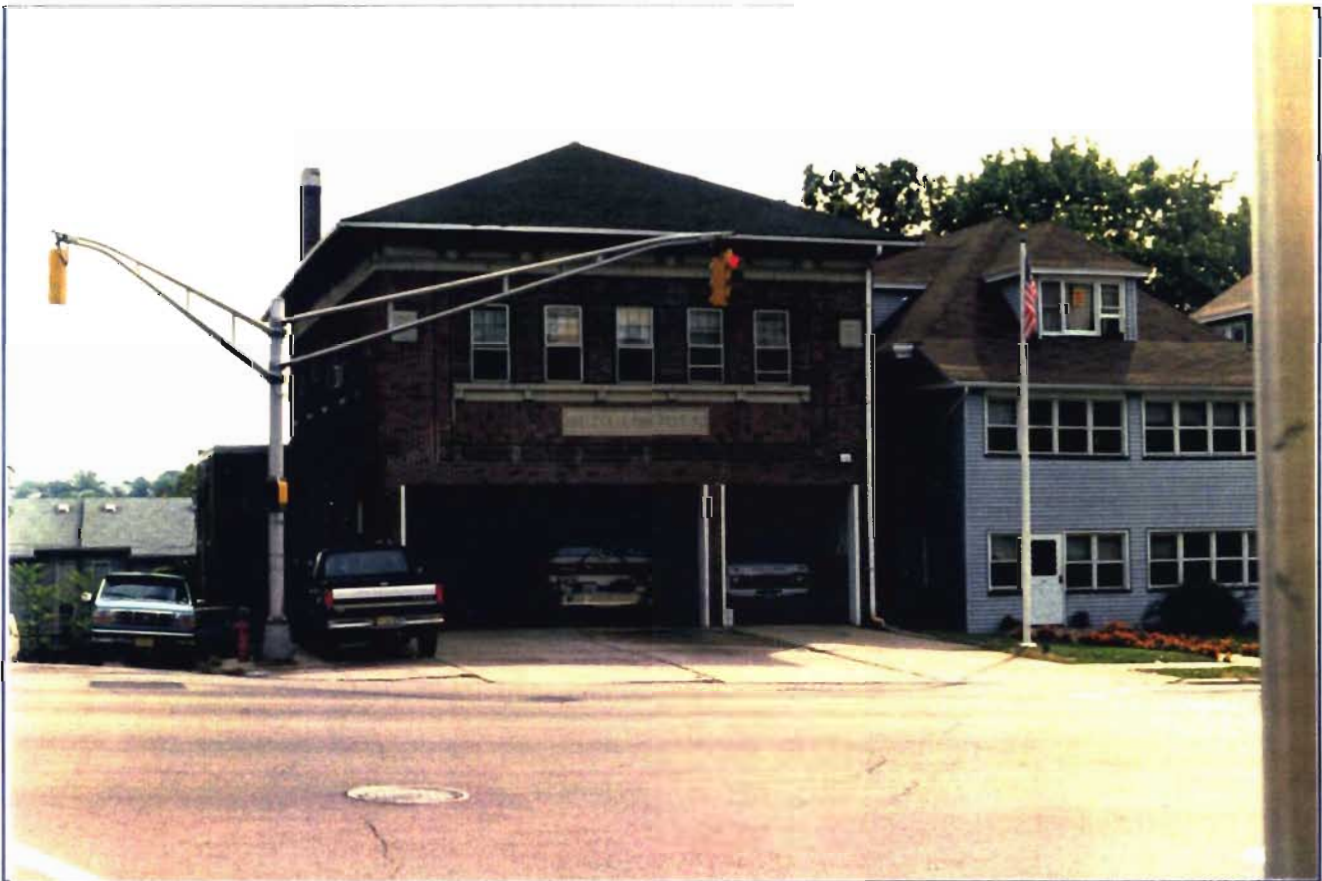
Photo F-3: Fire Station No. 2, Washington Avenue at Division Avenue.
